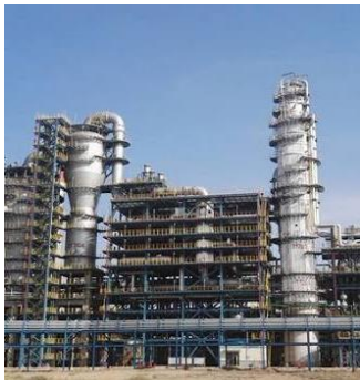
Methanol-to-olefins industrial plant (China)
