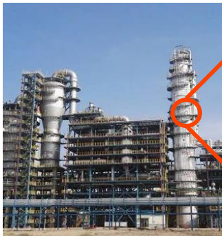
Methanol-to-olefins industrial plant (China)
